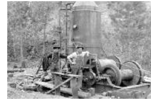
Donkey engines came in many different styles like this double-drum donkey. They could relocate under their own power by being tied to trees and winning themselves forward, even though they weighed about 10 tons. It must have been something to see them in operation....rumbling, belching monsters in the woods!
